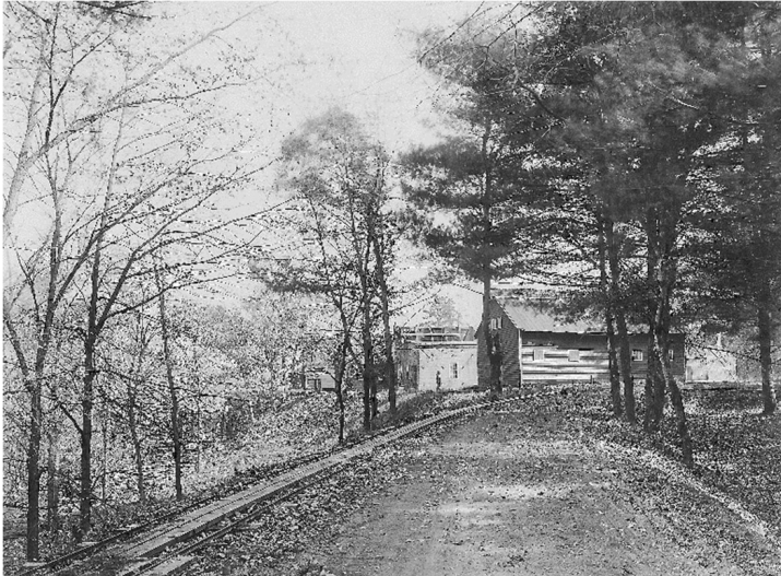
View of the New Works with the short rail to the left of the road where powder was transported between production buildings.
